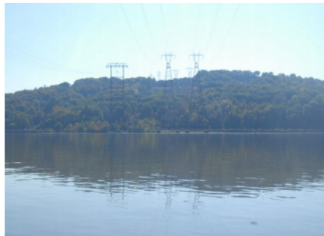
Easterly view of existing Hudson River crossing, Athens, N.Y. (Source: New York Department of Public Service)
