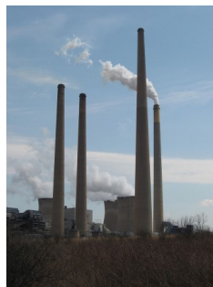
Homer City Generating Station
